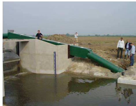
The new siphon type fish passage may be integrated in a fish guidance system.
